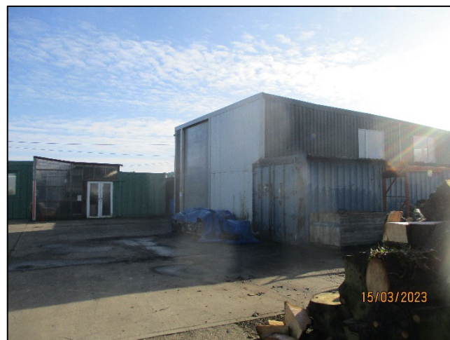
Showing building lying within the footprint
